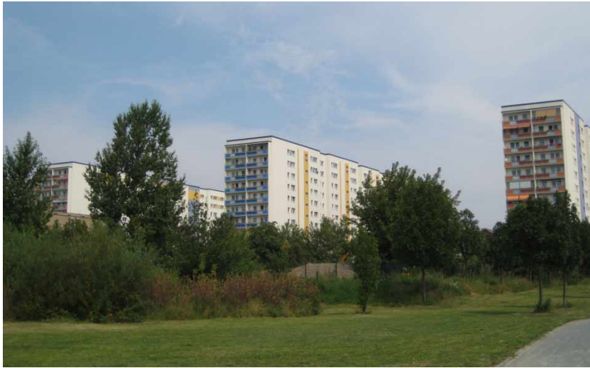
Figure 4 Apartment blocks in northern Marzahn. Source: Author.
